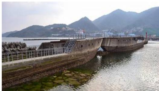
Fig. 13 Breakwater of Yasuura Fishery Port Constructed by No.1 & No.2 Takechi Maru
