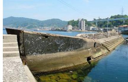
Fig. 8 Towing Concrete Tanker as Breakwater
