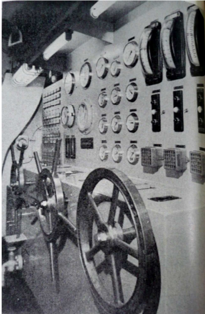
1 1) W43-11 UNIVERSE CONVEYOR Engine Control Room
