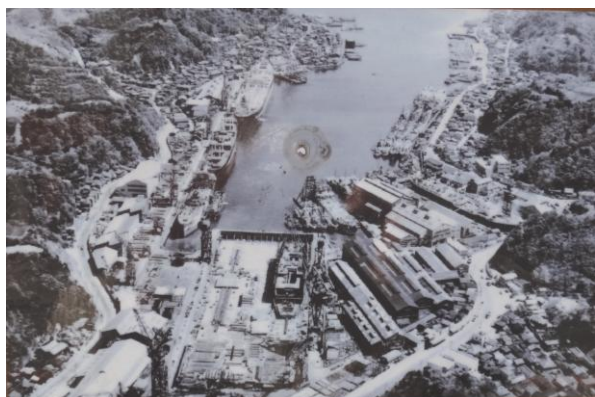
Fig.3 Photo of Uruga-dock around the year of 1950,taken from the outdoor notice by the author. Two cradles can be seen in the center. The right hand side of the two was used for the launching of Nippon Maru(II). There is the Uruga-station outside the bottom of this photo.
