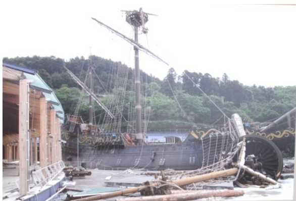
Fig.7 Photo from the panel showing the disaster area. Front spars and circular structure will be the broken mast by strong winds after the great earthquake on Mar.11'2011
