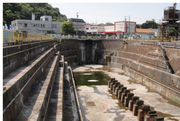
Fig.4 Looking toward the dock front of old Uruga Ship Yard (photo by author in 2016)
