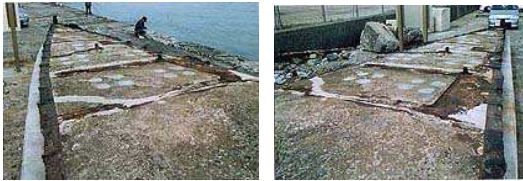
Photo 3 The top surface of destroyer (YANAGI) is photographed to the bow direction (corrosion / damaged) [cited from Ref. 3]
