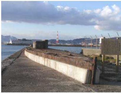
Photo 2 Whole view of destroyer (YANAGI) constituting a warship breakwater (GUNKAN-BOUHATEI) [cited from Ref. 3]
