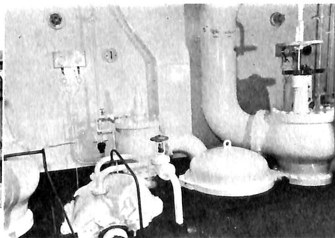
MAIN PUMP ROOM
