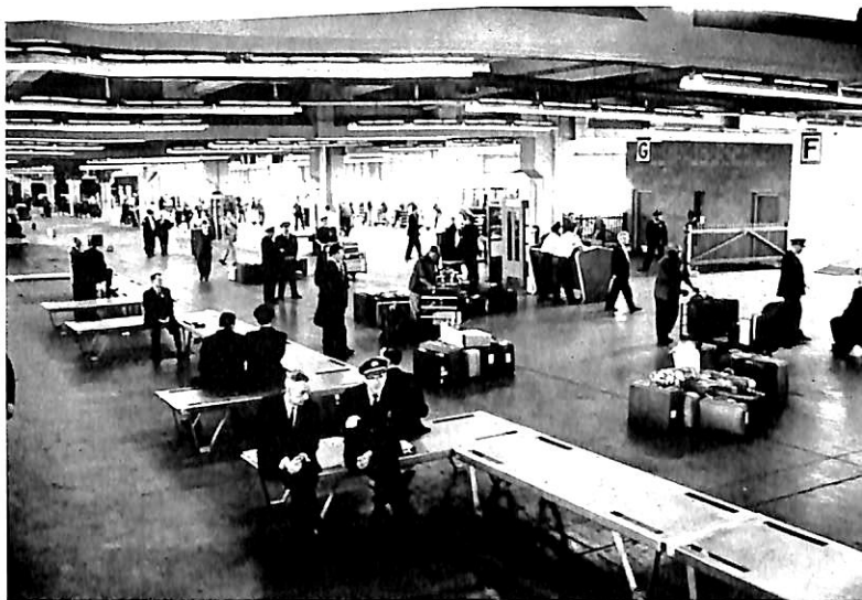
Passenger shed areas
