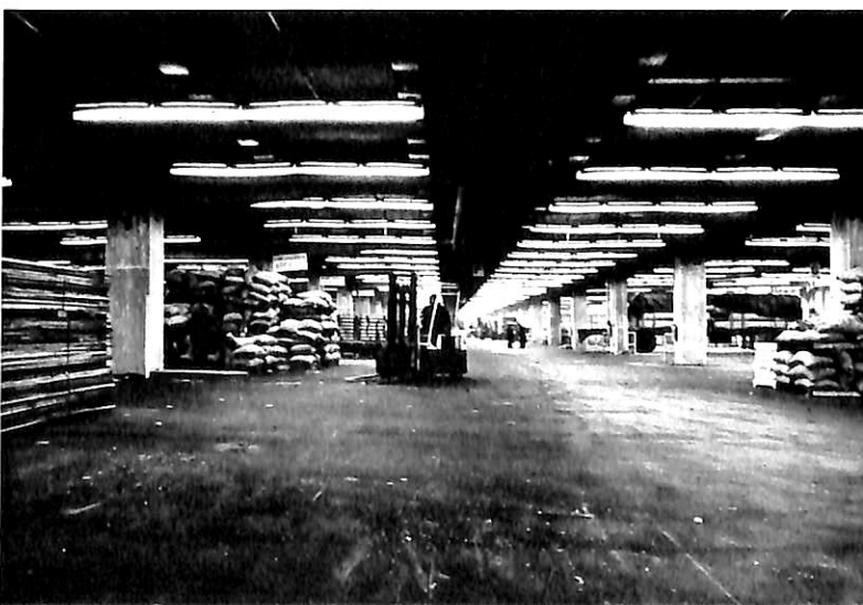
Cargo shed areas
