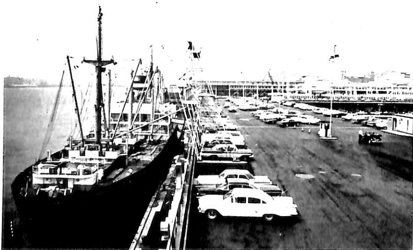
Open a'r roof deck (3rd. level) for parking 725 automobiles and 2nd. level truck court can accommodate 350 cargo vehicles, besides, 90 trucks are accommodated at the three sided loading dock
