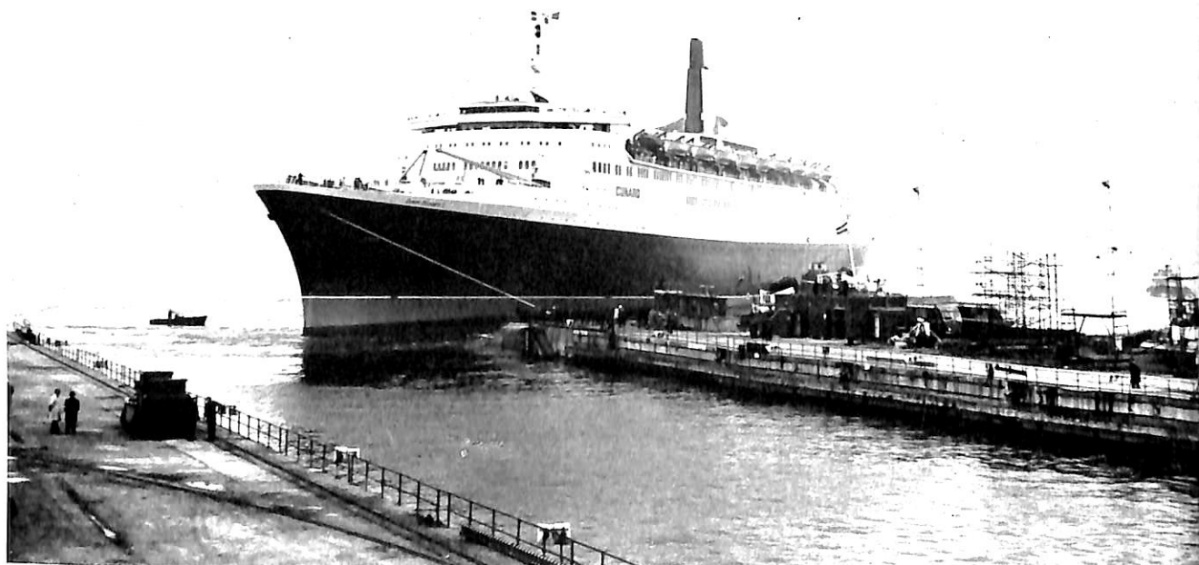
View going near to enter the dry dock
