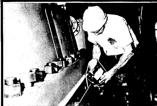
CHOCKFAST ORANGE 610TCfの注入作業
