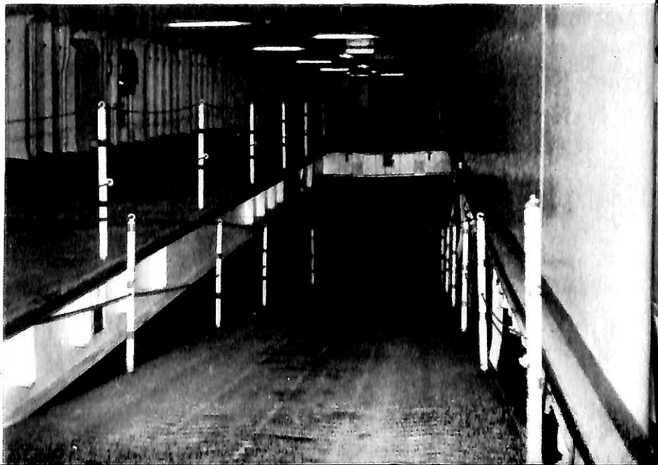
Driving Ramp for cars from Platform Deck to Upper Car Deck AURELLA
