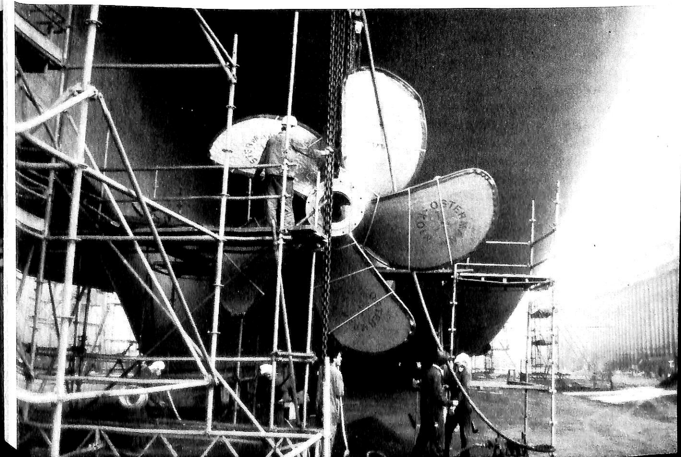
One of propellers fitting to shaft
