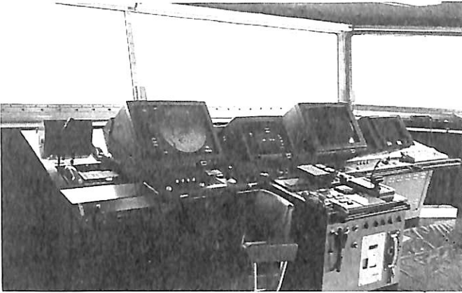
▲ IBS (Integrated Bridge System)
