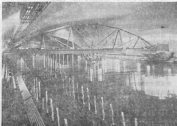
図 2-4 An indoor view of the Basin
